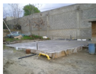
Here is the foundation to the Luciano's House.
